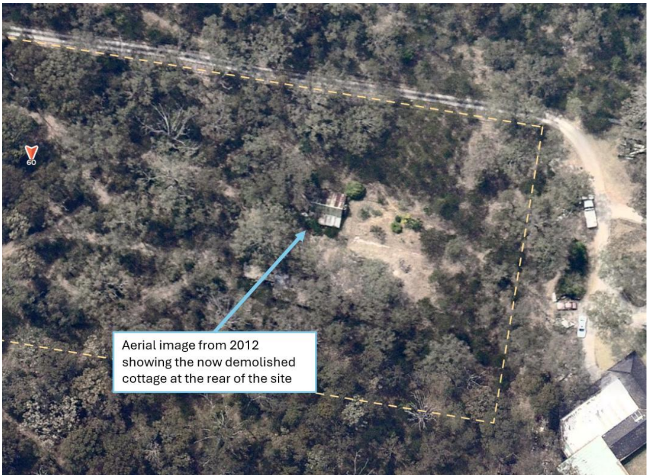
Figure 2 Aerial image of the rear of subject site showing the now demolished cottage (source: Nearmap)
